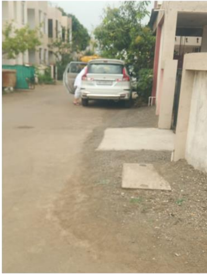
Covered Drain along the road - Sinnar
