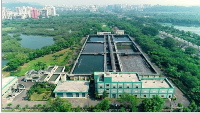
Sewage Treatment Plant
