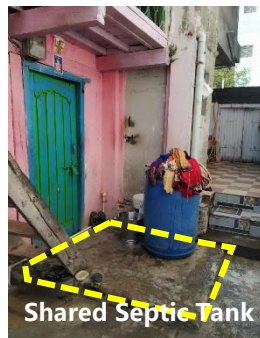
Khopoli - Shared septic tank in connected to 25-30 toilets
