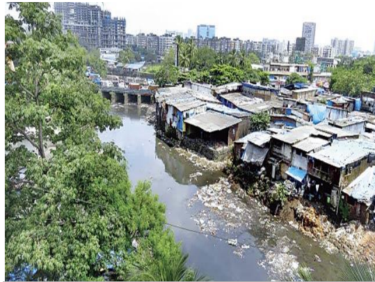
Drains outfall in River
