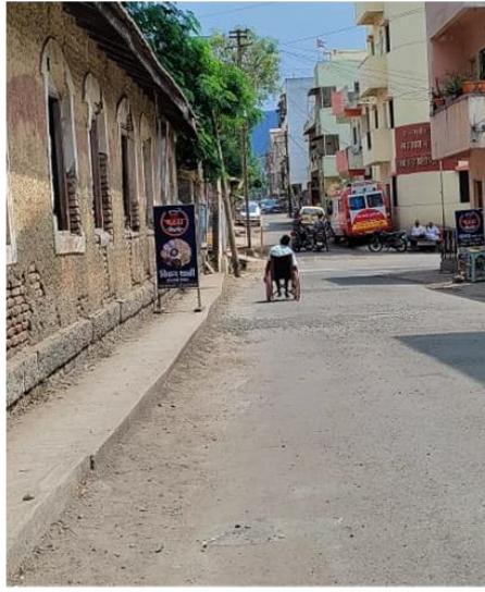
Covered Drain along the road - Wai
