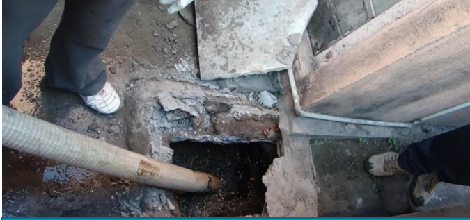
Emptying when the tank is full
