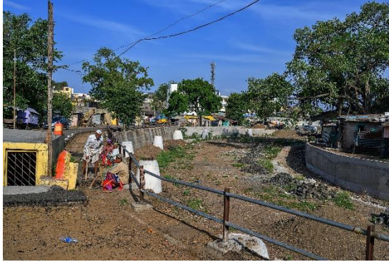
Interceptor and diversion drains
